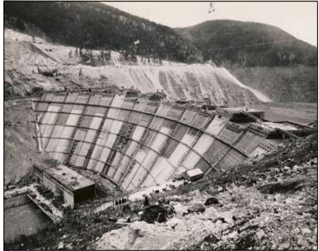
Hungry Horse Dam under construction.
